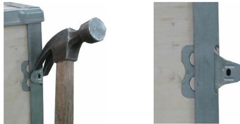
Figure 2-2 Straightening the hooks
