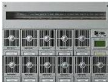
Original system with standard efficiency rectifiers
