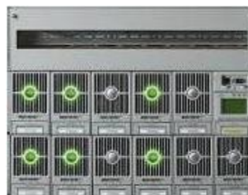
System upgraded with eSure high efficiency rectifiers required for normal load
